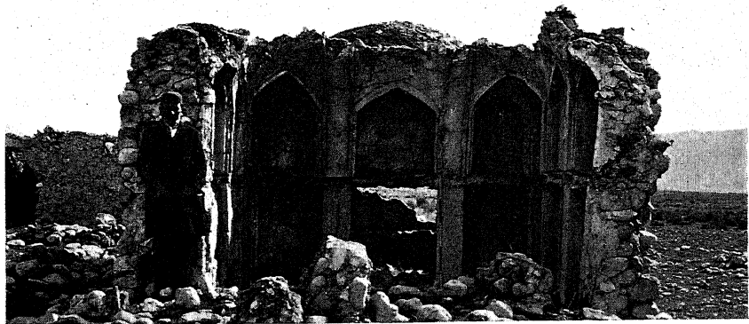
26. INTERIOR OF RUINED HOUSE AT AULISH, TĀSHĀN
